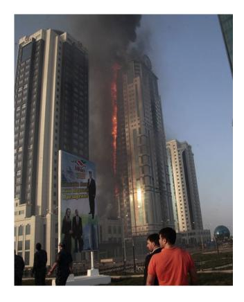
Upward fire spread with an inclined front
