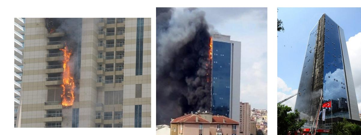
Upward vertical fire spread
